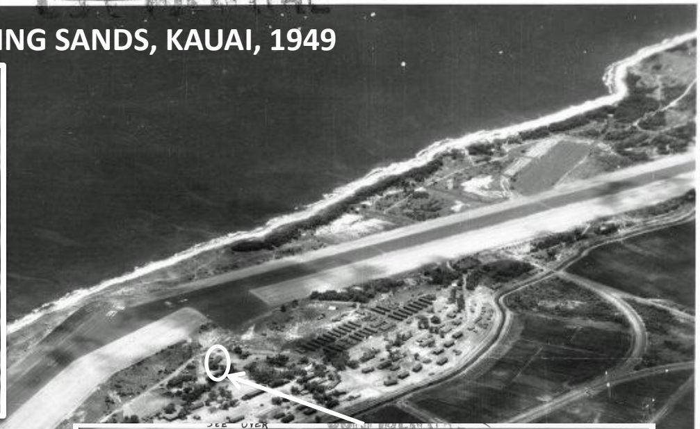
Carpentry Shop inside Motor Pool Area
