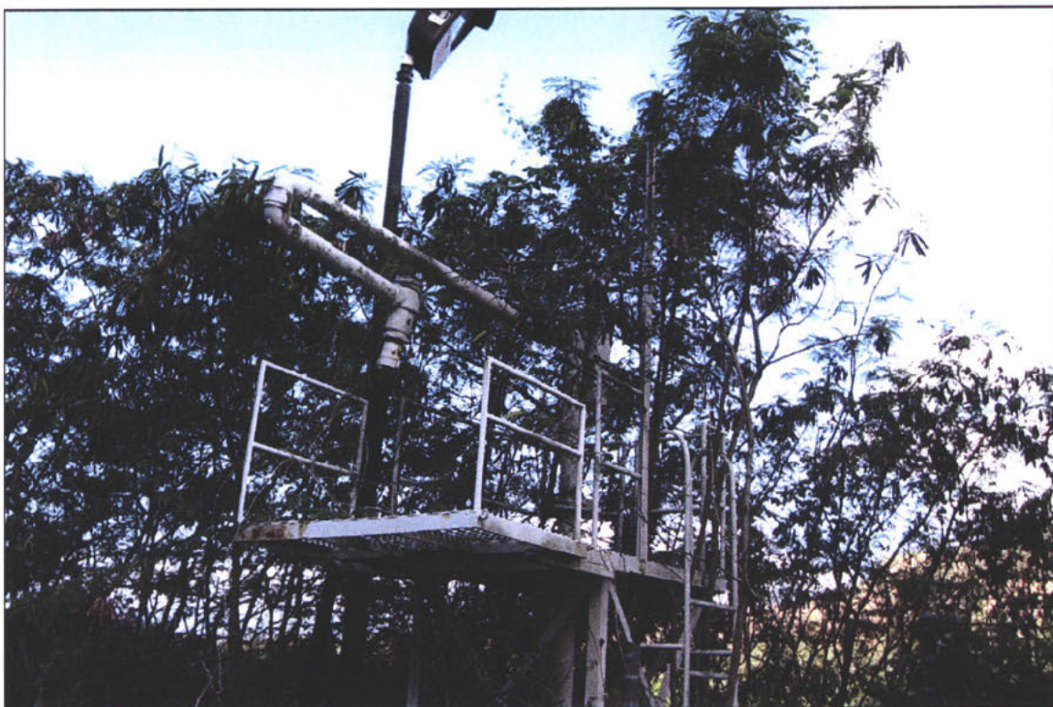
Photo No. 8: Truck-loading rack.
