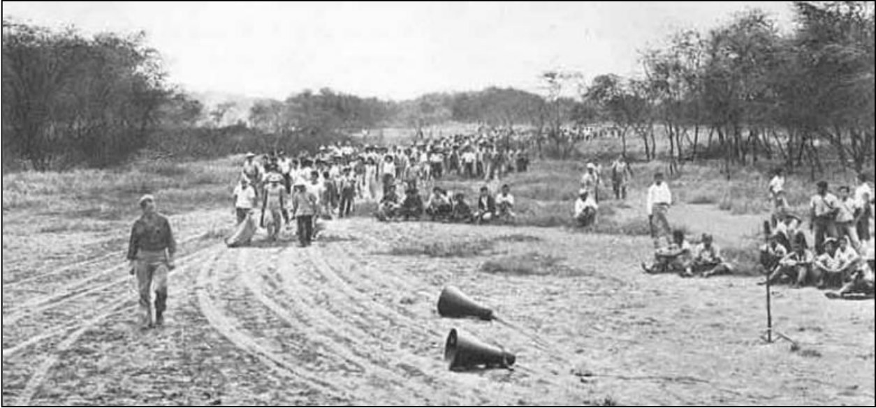
Figure 3.19. A photograph, taken in the early months of World War II, documents the arrival of the Keawe Corps for a clearing project at Barking Sands. Photograph from World War II on Kauai (Klass ca. 1970).
