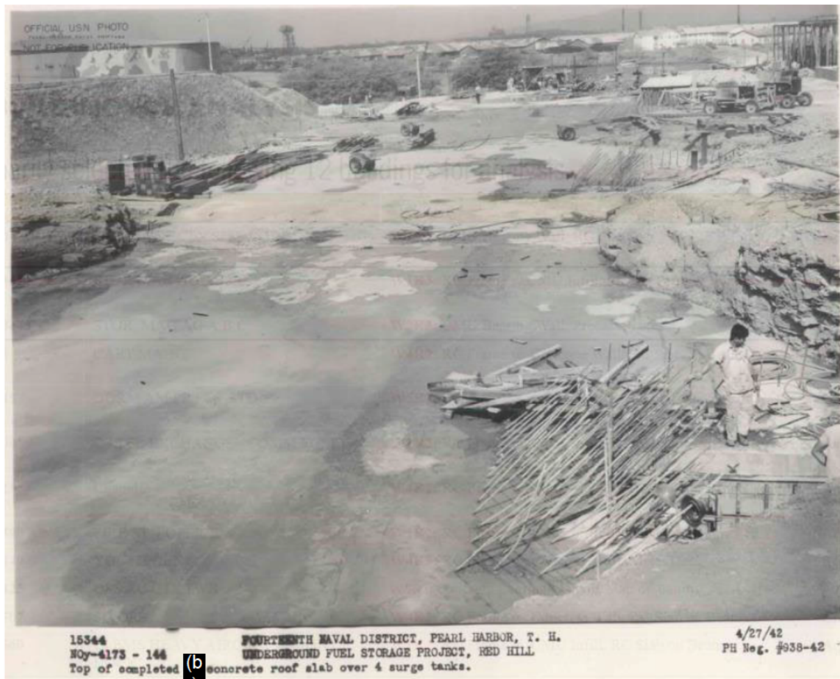
Figure 3 – Top of Completed 1 ft Thick Concrete Roof Slab over Four Surge Tanks
