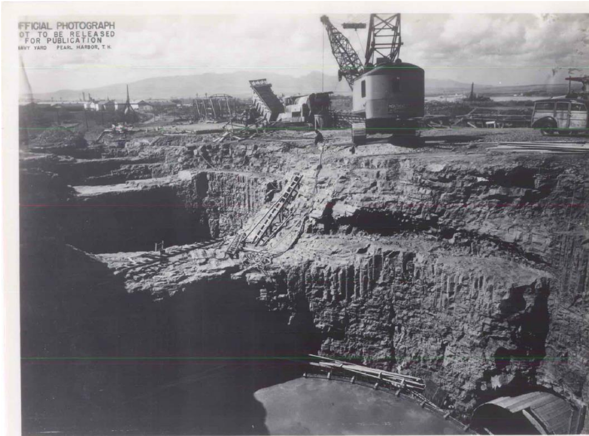
Figure 2 – Excavation from the Volcanic Tuff Rock Formation During Construction
