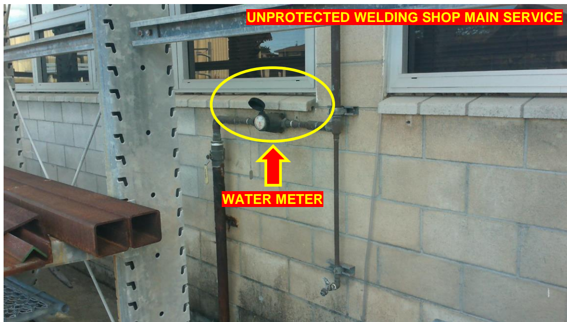
Figure 5-2 Priority Group 1 Example – Reduced Pressure Zone Assembly for Unprotected Service Connection
