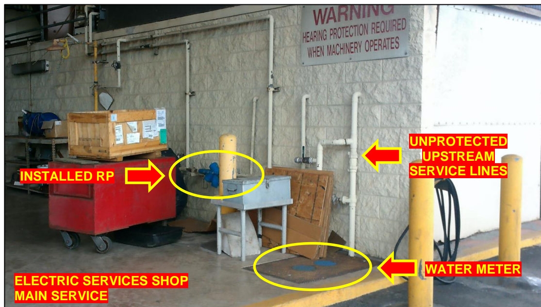
Figure 5-4 Priority Group 1 Example – Reduced Pressure Zone Assembly Relocation
