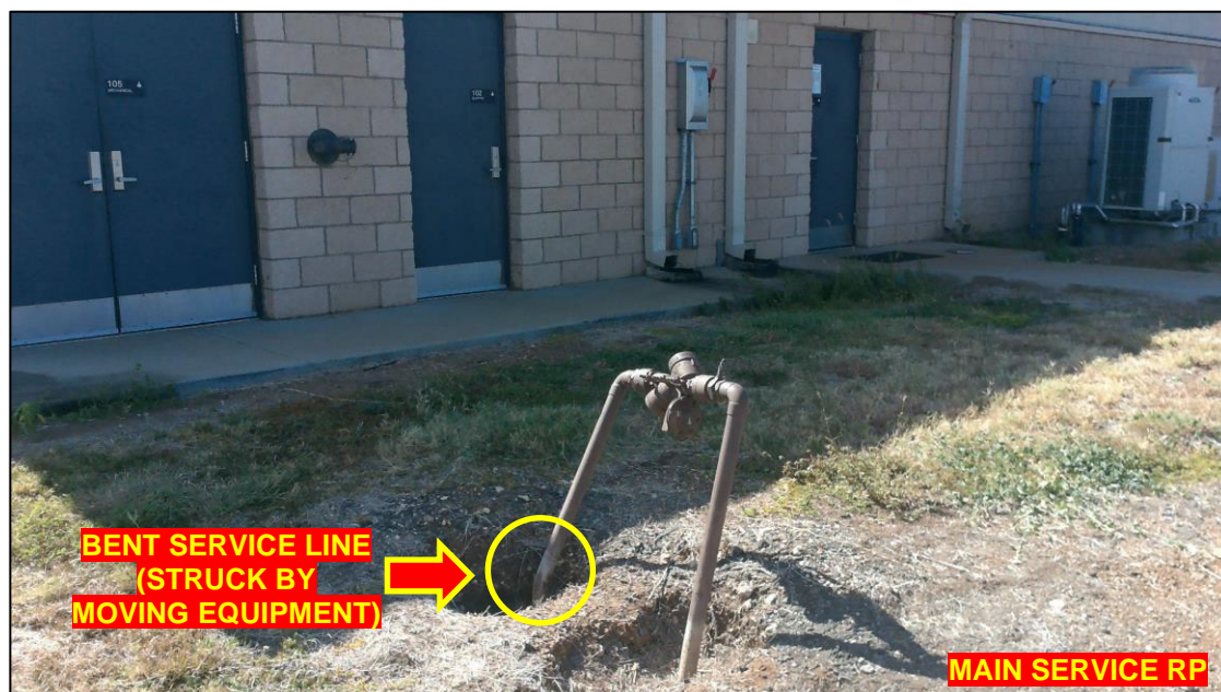
Figure 5-16 Priority Group 5 Example – Repair Bent Pipe
