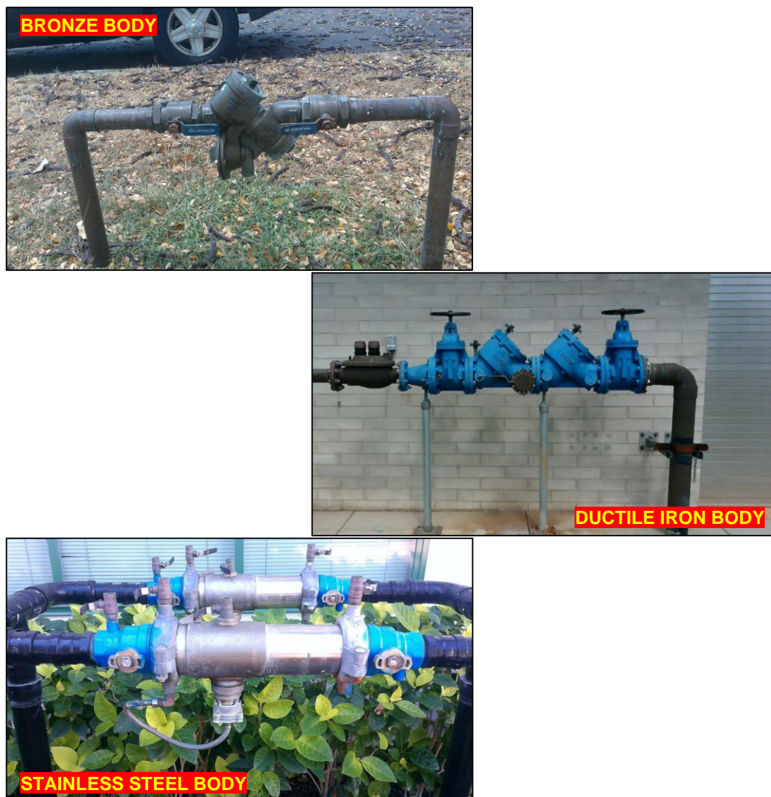
Figure 3-8 Reduced Pressure Zone Assembly Examples
