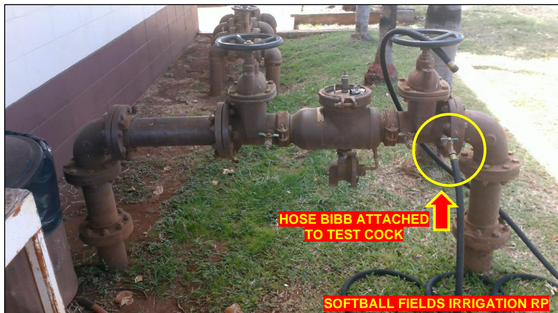
Figure 5-13 Priority Group 4 Example – Remove Improper Connections to Device
