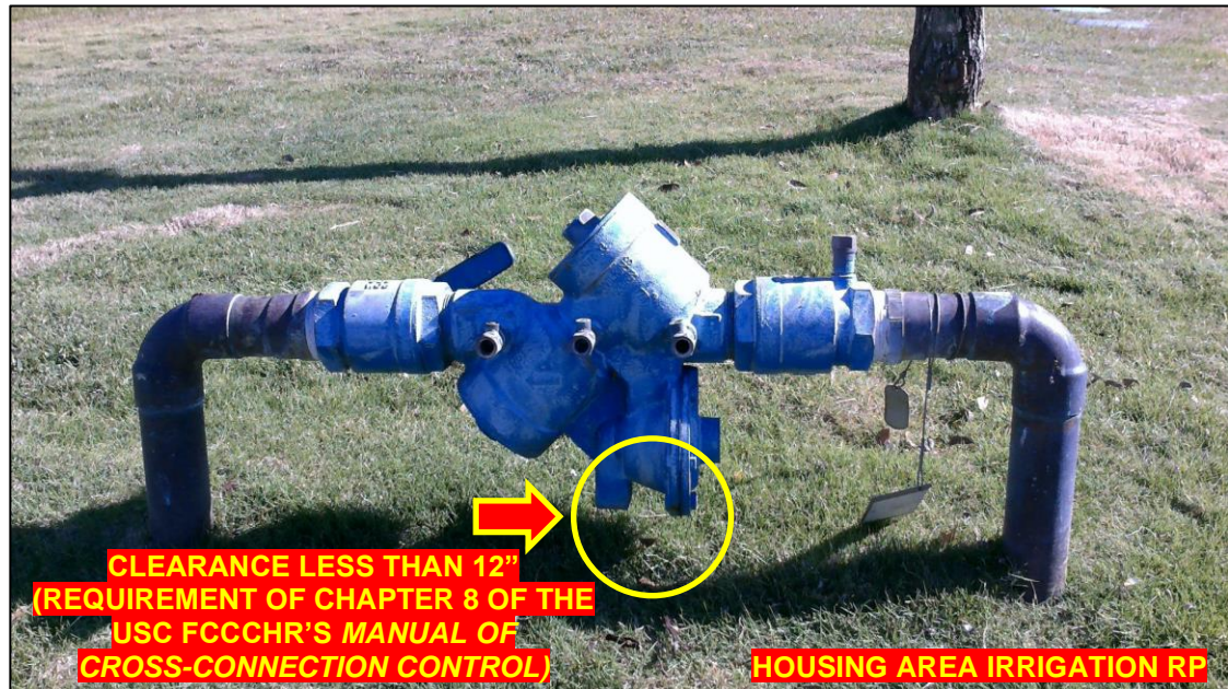
Figure 5-10 Priority Group 4 Example – Raise Backflow Prevention Device Position
