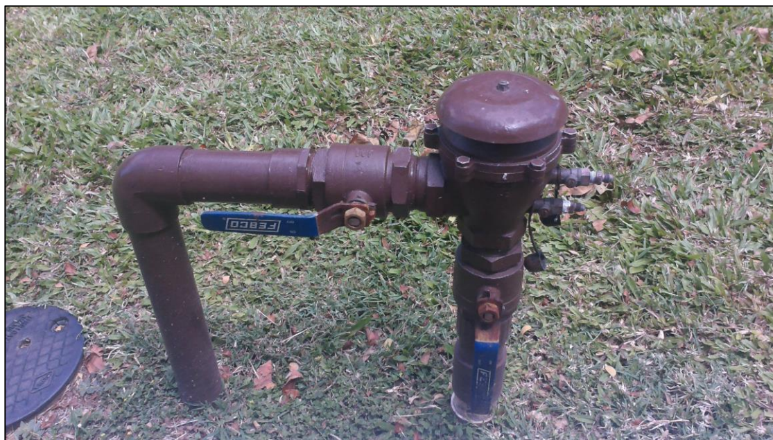
Figure 3-9 Pressure Vacuum Breaker Example
