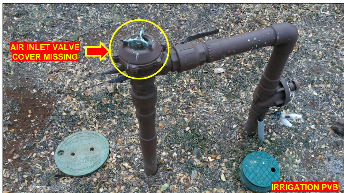
Figure 5-19 Priority Group 5 Example – Replace Missing Pressure Vacuum Breaker Air Inlet Valve Cover
