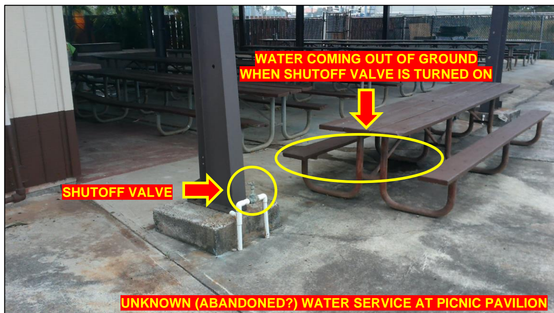
Figure 5-14 Priority Group 5 Example – Cap Pipe
