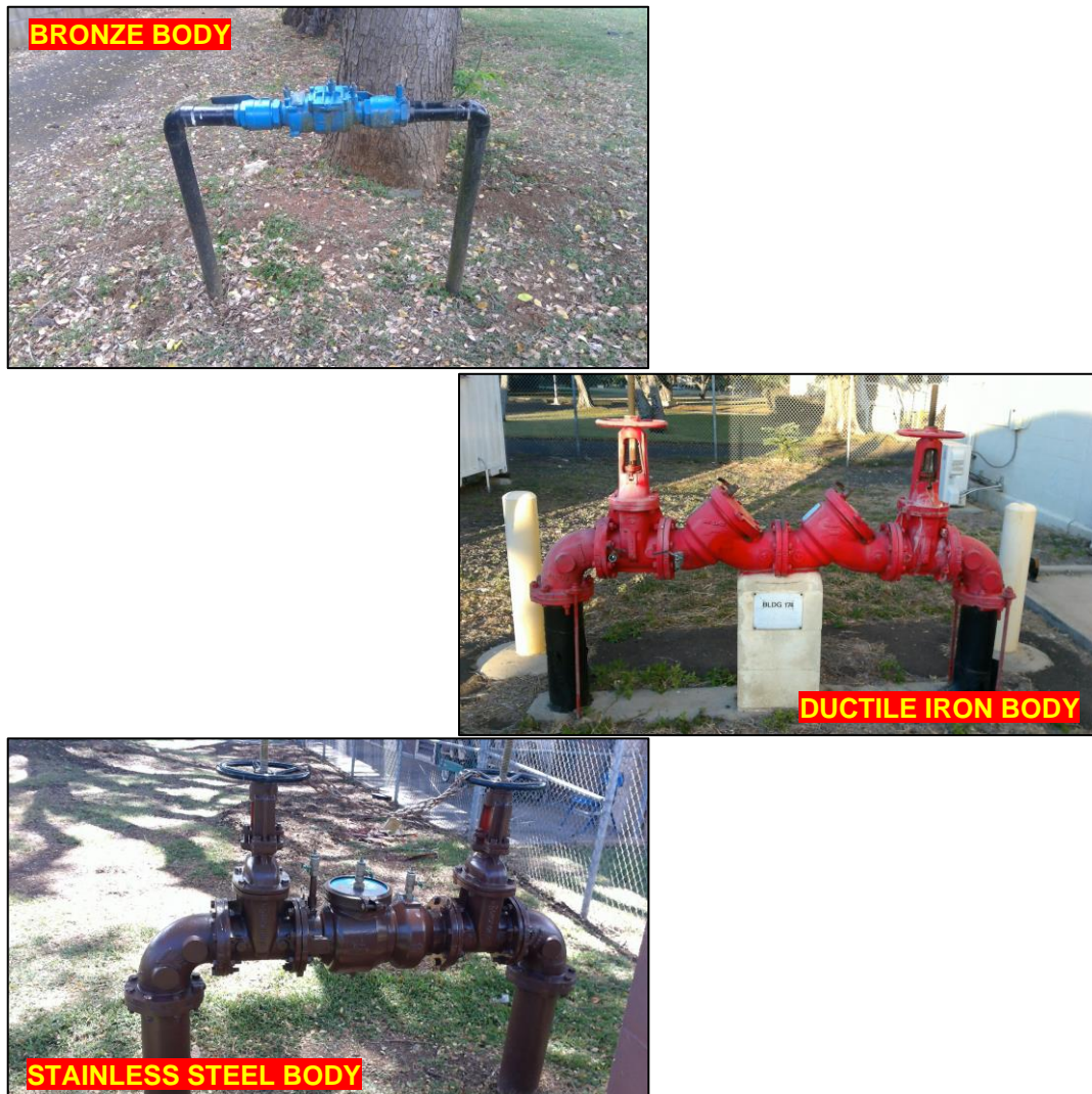
Figure 3-10 Double Check Valve Assembly Examples
