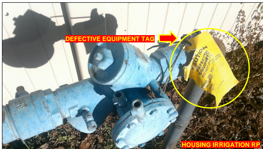
Figure 5-17 Priority Group 5 Example – Repair Broken Backflow Preventer Device
