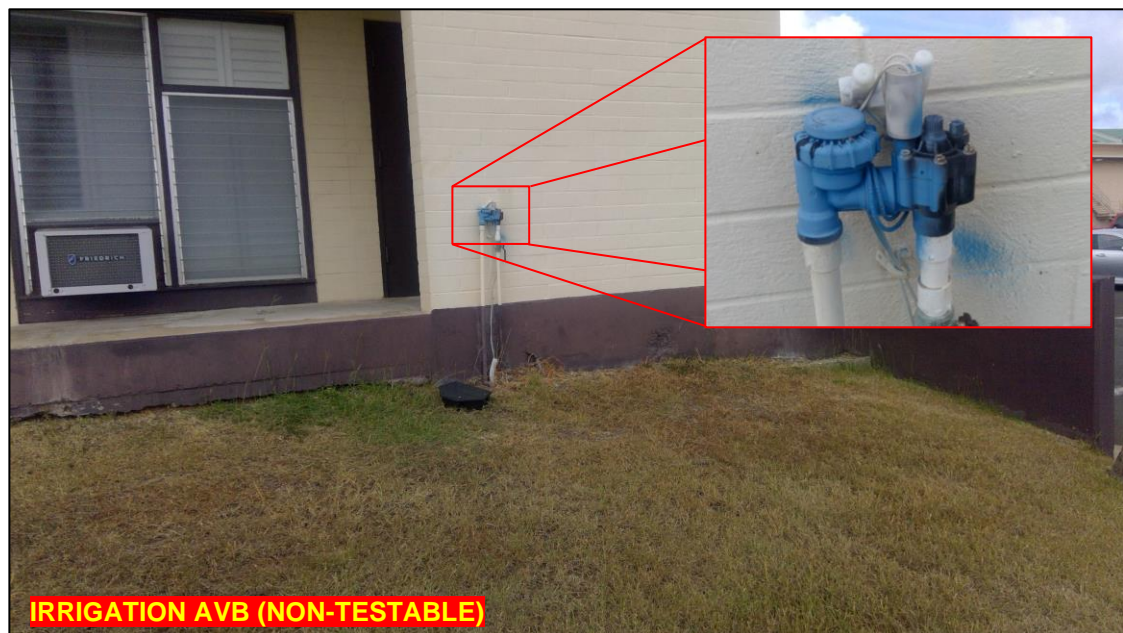
Figure 5-6 Priority Group 2 Example – Replace Air Vacuum Breaker with Pressure Vacuum Breaker
