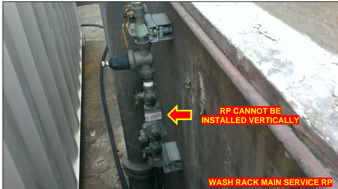
Figure 5-12 Priority Group 4 Example – Reposition Reduced Pressure Zone Assembly from Vertical to Horizontal Position
