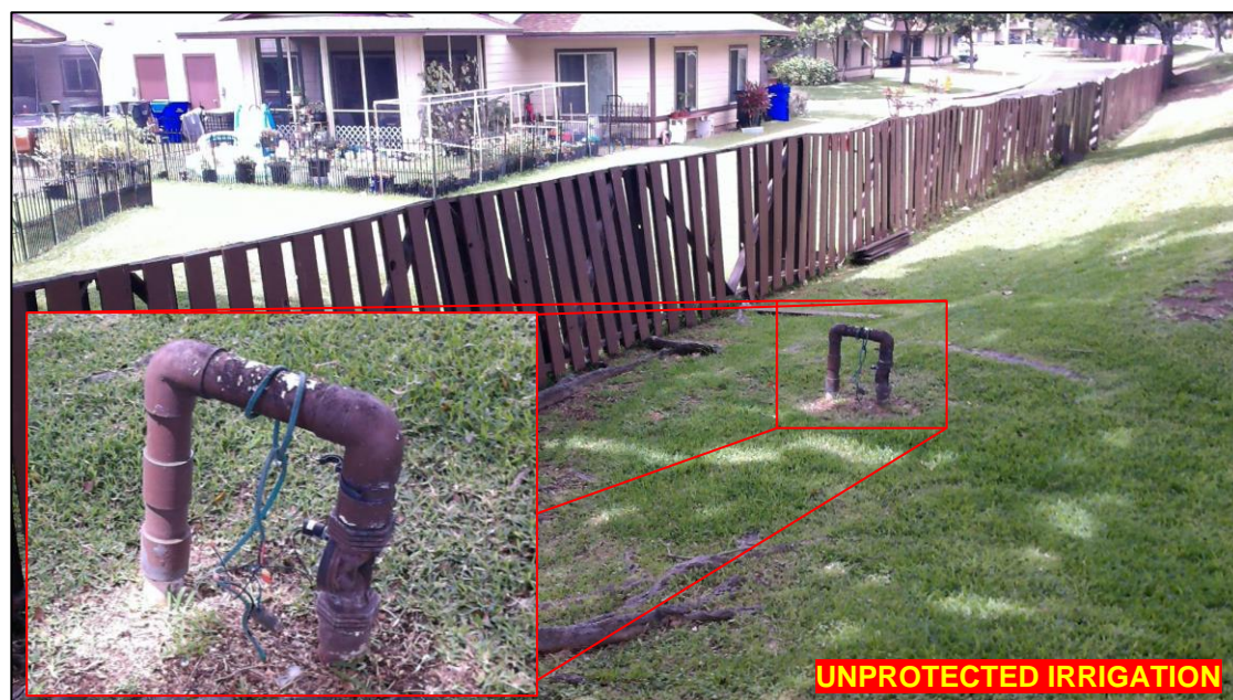
Figure 5-3 Priority Group 1 Example – Pressure Vacuum Breaker for Unprotected Service Connection
