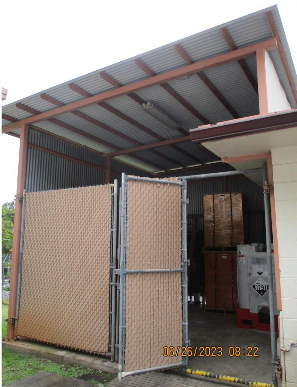
**Figure 1.** Storage space for totes of NaOCl solutions used for disinfection at Waiawa Shaft
