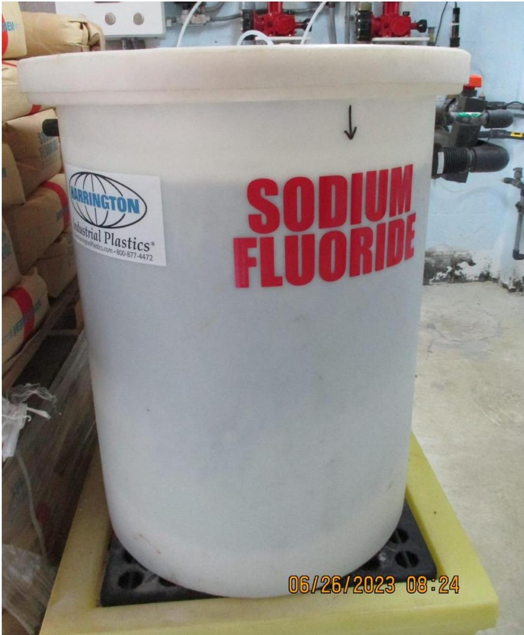
**Figure 9.** NaF solution for injection inside Building S-72
