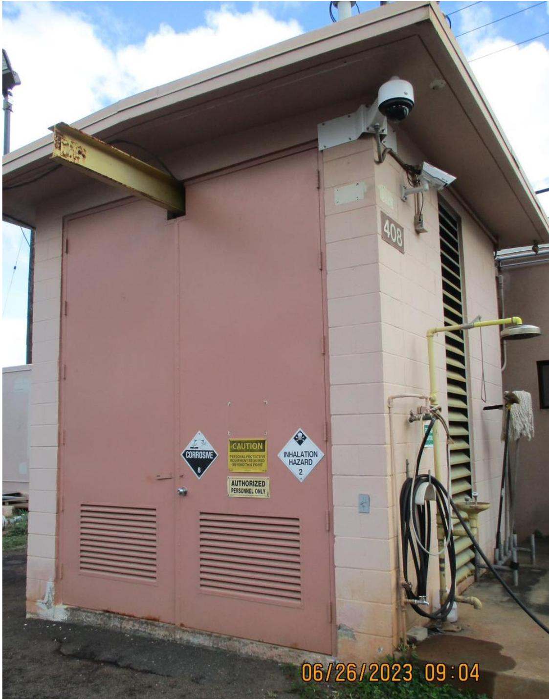
**Figure 15.** NaOCl storage and injection room at Aiea-Halawa Shaft (Building 408)
