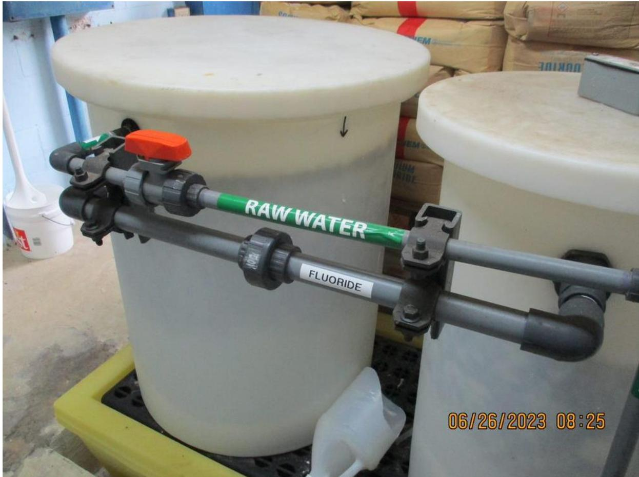
**Figure 10.** Connection lines for NaF and raw water inside Building S-72
