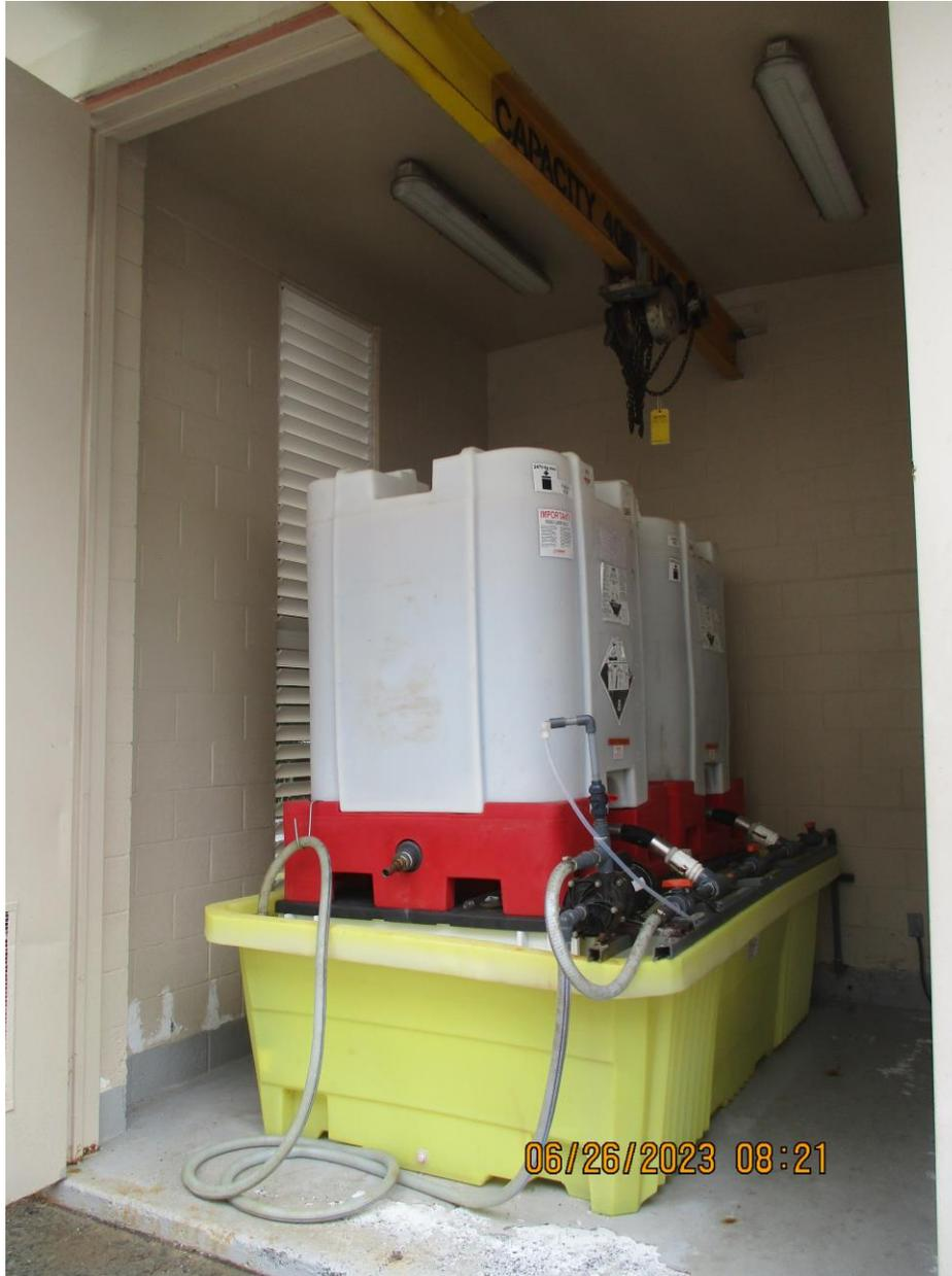
**Figure 3.** Pump room for NaOCl in totes with secondary containment (Inside view of Building 75)
