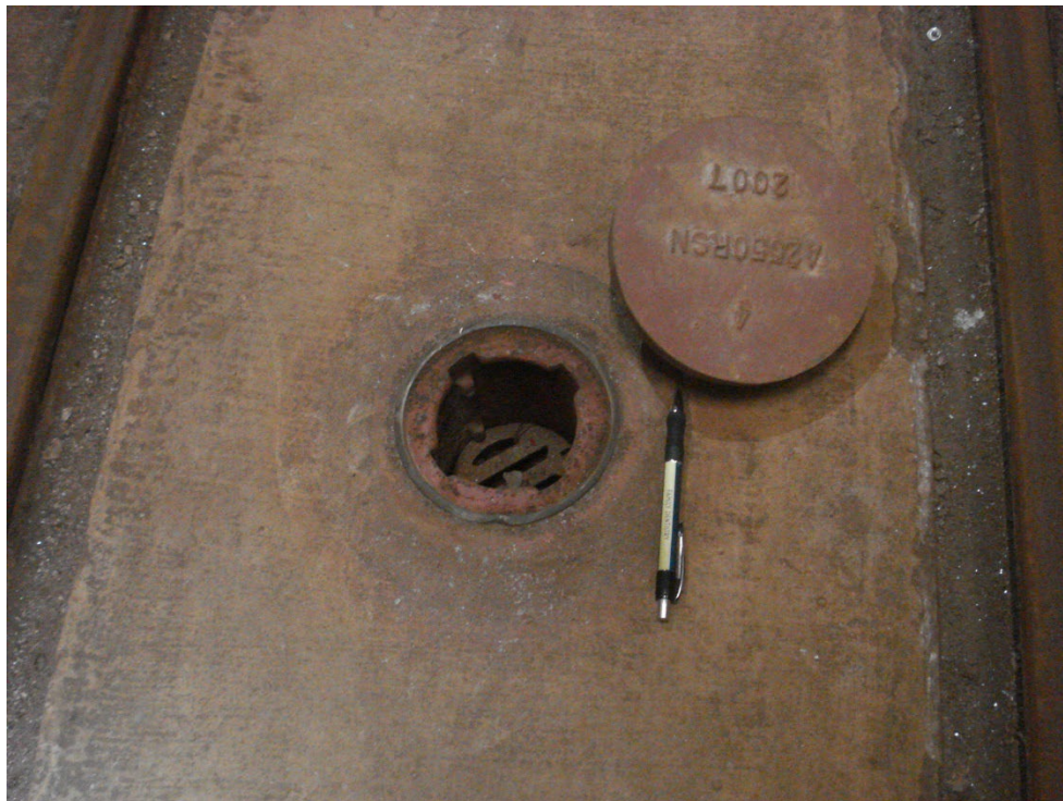
Figure 33: Drain covers with machined flat seal were caulked closed in Oct 2022.
