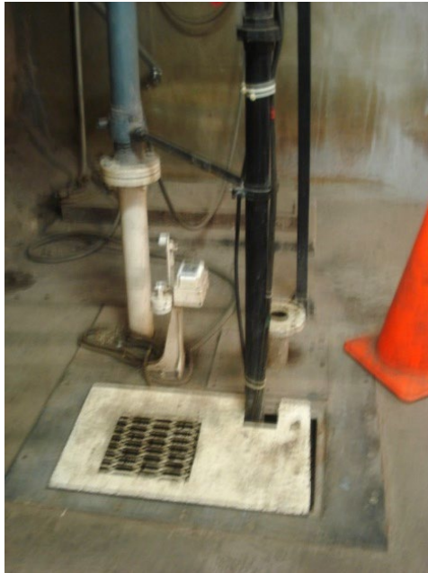
Figure 22: Sump and its vertical pipes have been sealed with rubber sheeting and caulk
