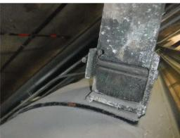
A30) One joint harness with gap noted on the dresser coupling at the large are no deflection rings and adapters on the harness lugs. Note: lugs are installed
