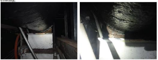
**Ке**fегелсе: І, **Long-Term** around the 7 o'clock position. Size could not be verified. That appears to be a dent underneath the thick coating is limited. There is one location near encapsulated asbestos coating from . Inspection of the pipe in this area to about A6) Finding: The (5) (F-24) line a arrs to have some type of thick asbestos or bitumen
