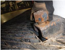
C22) **Finding:** The outlet side flange bolts he control valve on Pump (b) (3) are not fully engaged.
