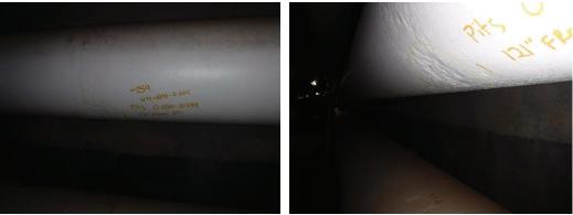
B34) Inactive pitting on at 6 o'clock. Corrosion Area is 3" x 2", Pit Depth is 0.114", Metal thickness on unaffected area is 0.383" - 0.387" resulting on a remaining metal thickness of 0.269" to 0.273".
