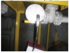
D8) Finding: Lack of thread engagement noted on the (b) (3) low suction pipe flange from (b) (3)
