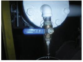
D10) **Finding:** Some minor staining noted on the bottom of the (b) (3) (A) (no active weeping noted). Note: See comment in Item D5 above about non-fuel related oily material related to epoxy coating curing.
