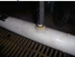
E2) **Finding:** Missing Teflon pad (metal-to metal contact) between pipe and support on Tank 20 FOR line in the trench past tank sampling line branch.
