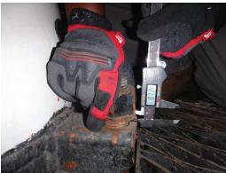
C2) **Finding:** Four loose joint harnesses were noted on the suction side of pump lower left = 0.200", lower right = 0.173", top right = 0.010", top left = 0.210" (See Notes above)
