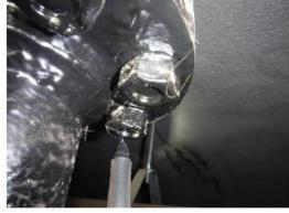
A17) **Finding:** There is a threaded fitting with brass (low melting) valve on top of the (b) (3) pipe at (b) (3). Note: these types of valves are not intended to be used on fuel systems. Some staining noted at the packing nut.
