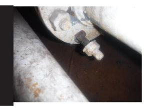
(b) (3) pipe with repair clamps at the FOR-Sump (S-E44) **Finding:** There are three locations on downstream of the isolation valve (shown with green arrow). The presence of these types of clamps indicate there were areas of compromised pipe sections at this location. A 6", 16" and 8" long full circumferential, single-section stainless steel repair clamp manufactured by Romac Industries is used with a 54section of the pipe. See next related inspection item.
