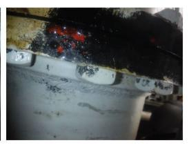
D6) Finding: Some staining noted on the om of the flange for the (b) (3) (A); just before pipe support (b) (3) (no active weeping noted). Note: See comment in Item 5 above about non-fuel related oily material.
