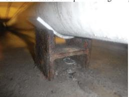
E5) Finding: Displaced pipe support on piping within trench between
