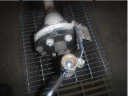
E8) **Finding:** Spray foam material used to 1 edge of AFFF Sump # 1. Foam material is in contact with pipe (Spray foam intent and function unknown).
