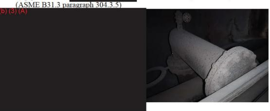
B42) Lack of thread engagement and one bolt missing a nut on flanged 6-inch branch fitting mounted on the 2 (F-76) line between . Note: the blind flange used also not ASME B16.5 rated/marked flange. It is a one-inch round plate with bolt holes (Plat thickness is 0.981" and appears to meet thickness required). ASME B16.5 NPS 6 class 150 blind flange has a minimum flange thickness of 0.940"
