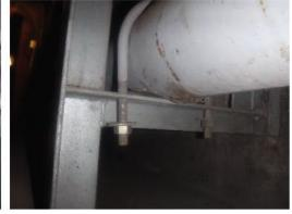
E52) **Finding:** Several locations with lose U-bolts, displaced Teflon pads, missing Teflon pads or loose hangers were noted. Some of the locations are summarized below with a full list to be provided in the report.
