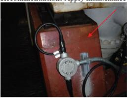
C12) Finding: Coating failure on pump casing on Pump (5) (3)
