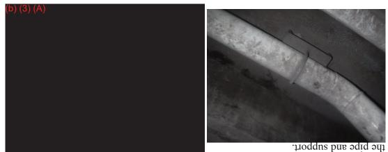
E34) **Finding:** Tank 4 sample lines are not ipped with skin valves positioned as close as practical to the tank shell (and or nozzle). This tank has approximately 30- of pipe between the tank and the first available isolation valve located at the sample manifold.
