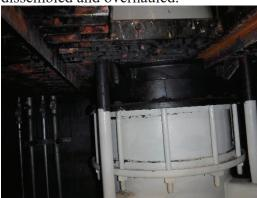
C8) **Finding:** Minor hairline crack noted on Pump (b) (3) pump pad. Note the hairline crack does not appear to be significant to warrant integrity concern and foundation pad is not exposed to precipitation were rebar corrosion is a concern.
