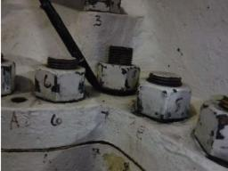
C6) Pump P-201 had a skillet installed on the discharge side of the pump nozzle. The assembled joint only had one gasket installed. Consider using two gaskets when installing spectacle blind or skillet to protect the flange face and contact surface from damage; particularly for flanges with serrated finishes (ASME B16.5 and ASME PCC-1-2019). Similar condition noted on P-205.
