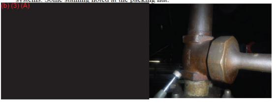
A20) Dresser coupling to Tank 14 is missing the deflection ring on the cap noted between the washer and harness lug.
