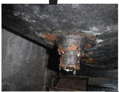
E.61 Coating failure and surface corrosion at threaded LPD (at
