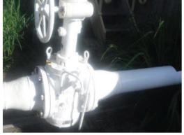
E63) The DBB valve (outside of the secondary containment of Tank 311) has one loose fastener. Note: Tank 311 has cathodic protection and fasteners with insulating
