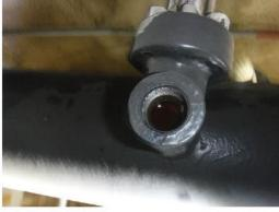
ith a drain valve in-leu of a plug. The end of the valve A4) Finding: The DBB valves are equipp is not secured with a pipe plug. This was noted on Tank 16 (b) (3) DBB), Tank 15 (b) (3) DBB), Tank 10 ((b) (3) DBB), Tank 9 (b) (3) DBB), Tank 8 (b) (3) DBB), Tank 7 (b) DBB), Tank 6 (b) (3) DBB), Tank 4 (b) (3) (A) DBB), Tank 3 (b) (3) (A)
