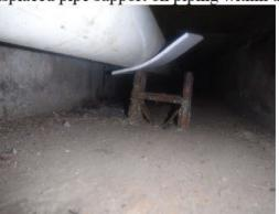
E6) Displaced Teflon pad pipe support within trench at (Photo)
