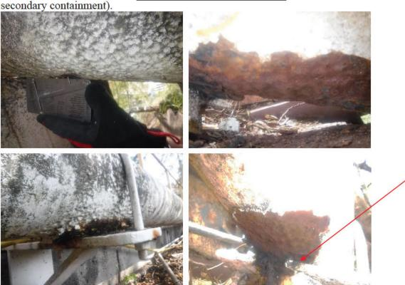
E61) Finding: Excessive vegetation around pipe (section of FOR pipe to (b) (3) (A)
