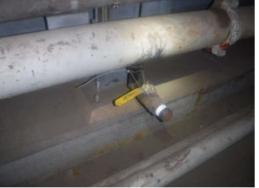
E56) A LPD with missing plug and a ball valve that is not locked-out was noted on the FOR line beneath ADIT 3 staircase (note: facility personnel corrected this finding).
