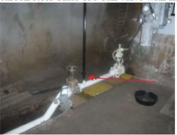
E21) **Finding:** (b) (3) (A) has one fastener that is not fully engaged.
