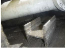
E19) **Finding:** Tank 16 sample lines are not equipped with skin valves positioned as close as practical to the tank shell (and or nozzle).
