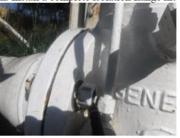
E65) **Finding:** The (b) (3) (A) valve (out of the secondary containment of (b) (3) (A) does not have a complete insulating flange kit (IFK). The gasket used does not appear to be insulating type and has one missing insulating washer. Additional test required to determine if IFK is functioning properly. NOTE: (b) (3) (A) and the segment of buried FOR piping outside of are protected by two sperate galvanic cathodic protection system.
