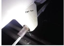
C26) One loose joint harness on the suction side of the joint harnesses of Pump P-205 (this is the same dresser coupling with the missing nut). Gaps measured between harness lug and nut were: Upper left = 0.250". lower left side = 0.275". (Facing pump)
