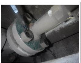
E55) **Finding:** There is a 2- LPD and 74 ch HPV (b) (3) (A) The LPD is missing a camlock cap, and there are two bolts that are not fully engaged on the 2- LPD flange.
