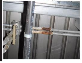
F13) **Finding:** There is a threaded nipple near tanks 11 and 12 installed with a <sup>3</sup>/<sub>4</sub>" ball valve. Note: There is staining/wetting on the lower threaded fitting. Location (b) (3) (A)
