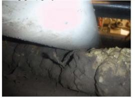
E9) The top of flange just before the FOR concrete pit; Sump 7 (near Door C) is covered with concrete to include side of the flange, face of flange, and fasteners.
