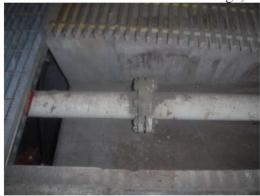
E10) FOR concrete pit; Sump 7 (near Door C), is not lined. Fuel contact water is dropped in this sump before it is picked up with sump pump to downstream segment of the FOR line. There is moderate sump floor-to-wall deterioration with periodic bubble formation
