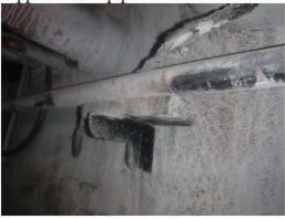
E14) Section for the FOR pipe from Sump 7 is threaded piping until it ties in to the Tank 15/16 FOR line.
