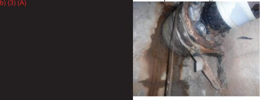
E59) **Finding:** There are moderate coating failure and corrosion on the FOR riser flange just outside of (b) (3) door. Note: there is a threaded (b) (3) fitting with a pressure gauge mounted on the flange.
