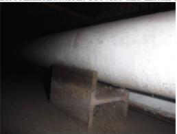
E41) Finding: Missing Teflon pad (metal-to metal contact) between pipe and support on FOR line
