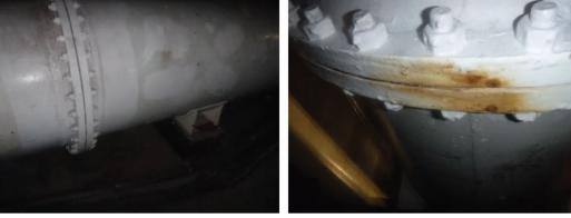
D13) Finding: Some staining noted on the bottom of the flange for the (some staining noted on the floor but no active weeping noted). Note: See comment in Item D5 above about non-fuel related oily material.
