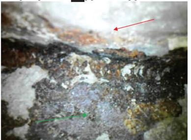
Red arrow is pipe and green arrow is the anchor plate/ring welded around the pipe. The plate/ring is approximately inches from the surface (near the middle of the bulkhead).
