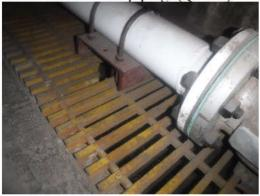
E33) Tank 4 sample lines are not equipped with skin valves positioned as close as practical to the tank shell (and or nozzle). This tank has approximately t of pipe between the tank and the first available isolation valve located at the sample manifold.
