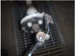
E8) Spray foam material used to seal edge of AFFF Sump # 1. Foam material is in contact with pipe (Spray foam intent and function unknown).
