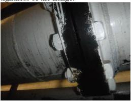
D7) Finding: There is a missing cap on a 1- ball valve that is mounted to the 4- low suction line at (b) (3) (A)
