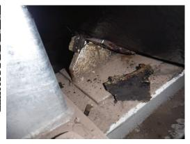
F18) **Finding:** There are moderate coating—lure and heavy corrosion at the pipe support I-beams The majority of the corrosion was noted at the base of the I-beams. Spalling concrete/broken grouting fill were also noted. These were identified on the second pipe support after Tank 19 (left hand side facing the tank), on the first pipe support after (b) (3) (A)
