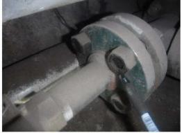
E54) There is a 2-inch LPD and <sup>3</sup>/<sub>4</sub>-inch HPV near The LPD is missing a camlock cap, and there are two bolts that are not fully engaged on the 2-inch LPD flange.
