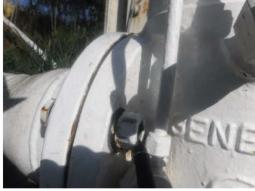
DBB valve (outside of the secondary containment of Tank 311) does not have a complete IFK. The gasket used does not appear to be insulating type and has one missing insulating washer. Additional test required to determine if IFK is functioning properly. Note: it may be practical to install ICCP on Tank 311 and remove the IFK to extend CP to the section of buried piping at ADIT 3 (review of the 2021 CP Report indicated the section of buried piping had ineffective magnesium anode).
