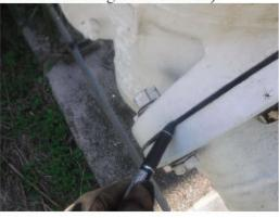
E65) The TRV bypass lines (QTY 2) at Tank 311 does not have a complete IFK. Only has insulating washer on the lower flange. The gasket used also does not appear to be insulating type.
