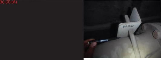
E50) Finding: Segment of tunnel piping from the constructed with mechanical coupling (Style 77 Victaulic joint). Some discoloration corrosion cell and staining were noted at the following joints located at (b) (3) (A)
