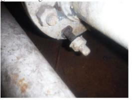
E46) The DBB on the sump pump discharge line before the strainer is missing a body cavity relief valve handle. The valve is also not plugged when not used.
