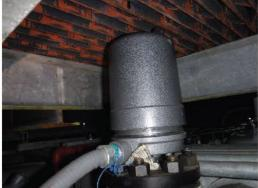
C30) The ½-inch discharge side pressure gauge threaded fittings have several areas of wetting/weeping around the threaded fitting on Pump P-208. Wet absorbent pads noted
