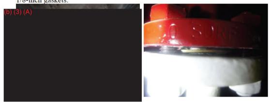
D12) Some minor staining noted on the bottom of the flange for the F-76 line from Surge Tank 4; just before pipe support F76-8 (some staining noted on the floor but no active weeping noted). *Note: See comment in Item 5 above about non-fuel related oily*
