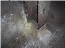
F19) **Finding:** There is a loose I-beam base plate anchor bolt at (b) (3)
