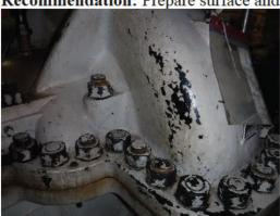
C13) Finding: The ½- valve (b) (3) (A) mounted on the suction side of the pressure gauge pipe on pump (b) (3) is missing plug and valve is non-lockable type.
