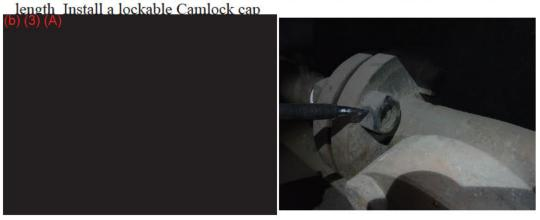
E56) **Finding:** An LPD with missing plug and a ball valve that is not locked-out was noted on the FOR line near (b) (3) (note: facility personnel corrected this finding).
