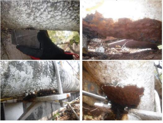
E59) There are moderate coating failure and corrosion on the FOR riser flange just outside of ADIT 3 door. Note: there is a threaded fittings with a pressure gauge mounted
