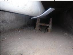
E6) Finding: Displaced Teflon pad pipe support within trench at
