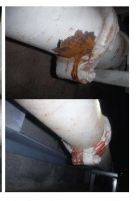
is damaged likely due to impact with displaced pipe support and U-bolt. E50)
