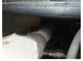
E36) **Finding:** There is a segment of unsupported (b) (3) (A) piping spanning (b) (3) at Tank 3 (Note industry standard is fourteen span for 1.5-pipe).
