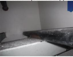
E17) **Finding:** The segment of the FOR and has four brass/bronze (low melting point) valves where the line ties in to Tank 15/16 FOR trench piping. This includes the temporary line that is attached to the F76 header pipe.
