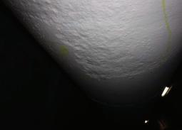
B36) Wood shim installed on (f-76) pipe between Teflon pad and concrete saddle in an attempt to correct lack of support at concert saddle # 193 (Between 0). Pipe is not fully and uniformly supported.
