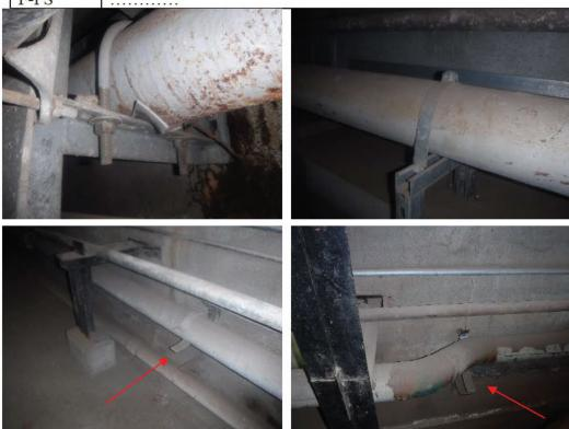
E52) Areas of total coating failure and heavy corrosion were identified on sections of the FOR line. Some of the locations are summarized in the table (note: some coating repair activity was noted during the inspection on some specific locations):
