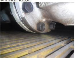
E24) **Finding:** Tank 15 sample lines are not equipped with skin valves positioned as close as practical to the tank shell (and or nozzle).
