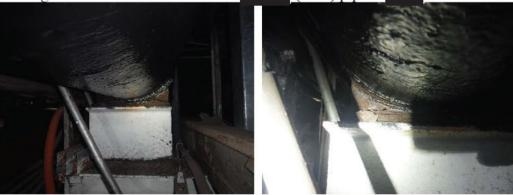
A5) The \_\_\_\_\_\_ (F-24) line appears to have some type of thick asbestos or bitumen encapsulated asbestos coating from \_\_\_\_\_\_ to about \_\_\_\_\_. Inspection of the pipe in this area is limited. There is one location near \_\_\_\_\_ 38 that appear to be a dent underneath the thick coating around the 7 o'clock position. Size could not be verified.
