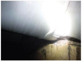
D2) Deteriorated grout noted at the bottom of the pipe support at Surge Tank 1 (just past the isolation DBB valve).
