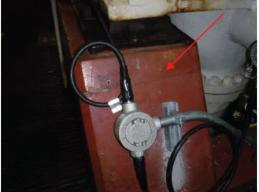
C12) Coating failure on pump casing on Pump P-202
