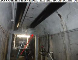
E37) **Finding:** Tank 3 sample lines are not to the tank shell (and or nozzle).
