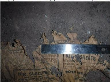
Note the piping and coating appears to be original to the facility. Same black coating noted on the newspaper. Reason for the paper is unknown but likely to seal the concrete form boards during construction.
