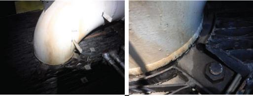
C33) Dresser lugs on Pump P-210 suction side are installed backward (this was also noted on the
