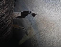
B33) Finding: Inactive pitting on (b) (3) (JP-5) line between (b) (3) (A) 10 o'clock. Corrosion Area is 8" x 8", Pit Depth is 0.050" - 0.135", Metal thickness on unaffected area is 0.226" - 0.234" resulting in a remaining metal thickness of 0.091" to 0.099". Reference: A/I, Mandatory
