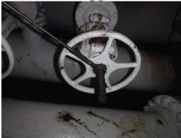
C45) There is DBB valve on the line (Valve # 232E2) with six studs that are not fully engaged. The stud is supposed to be engaged on the upper position of the DBB flange anywhere from 1.75 to 1.88 inches. Threaded engagement of only 0.25 to 0.75 inches where measured. Green arrow shows the available thread depth, the red arrow shows measured engagement depth of studs. (black dots marked with black Sharpie on the flange).
