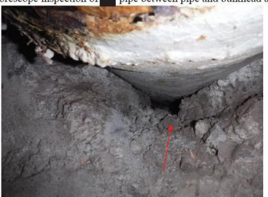
Space between pipe and the concrete bulkhead was used to perform borescope inspection of the cavity.
