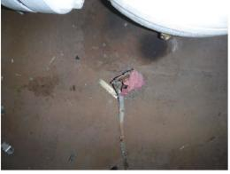
C36) Several brass/bronze fittings used on the fuel system (low melting point material). Gate Valve GI58I shown). Same for Valve GI58G, GI58H.
