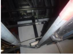
E15) **Finding:** Section of NPS 1.5 threaded FOR piping between (b) (3) (A) has three segments of unsupported piping measuring 23 ft, 22 ft and 20 ft respectively. Note: industry standard is nine-span for 1.5-spaper.
