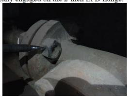
E55) A LPD with missing plug and a ball valve that is not locked-out was noted on the FOR line near (note: facility personnel corrected this finding).
