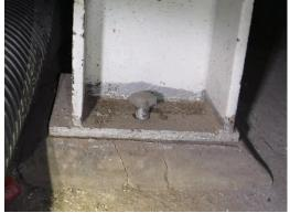
F20) **Finding:** There is an 18- dresser coupling joint and associated joint harness between S 25 just past the concrete penetration. Visual inspection did not reveal any deficiencies at this location. A slight tilt was noted and documented. Approximately a 0.9 ° tilt over a 36" span was recorded.
