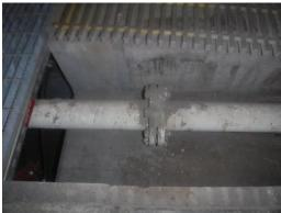
E10) **Finding:** FOR concrete pit; Sump 7 (near Door C), is not lined. Fuel contact water is dropped in this sump before it is picked up with sump pump to downstream segment of the FOR line. There is moderate sump floor-to-wall deterioration with periodic bubble formation from bottom the sump.
