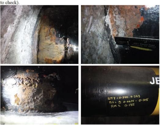
B46) Coating at the harbor tunnel consisted of bitumen with asbestos warp; sections with wax tape wrap and coating with lead and another hazardous chemical.
