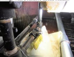
C31) **Finding:** One slightly loose joint harness was noted on the discharge side of pump (6) (3). Gaps measured between harness lug and nut were approx. 0.030" (enough for the rod and bolt to move laterally).
