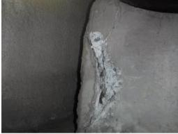
B47) **Finding:** Out-of-round/flat spot noted on the (b) (3) (JP-5) between (b) (3) (A) bell-weld (12 o'clock to 3 o'clock position).
