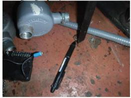
Several open conduits and sensor enclosures noted on pump C4) pump appears to be undergoing repair).
