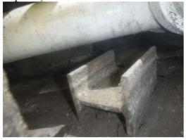
E19) Tank 16 sample lines are not equipped with skin valves positioned as close as practical to the tank shell (and or nozzle).
