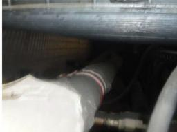
E36) Tank 3 sample lines are not equipped with skin valves positioned as close as practical to the tank shell (and or nozzle).
