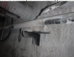
E14) **Finding:** Section for the FOR pipe ff Sump 7 is threaded piping until it ties in to the Tank 15/16 FOR line.
