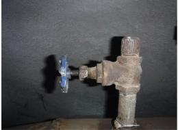
A18) Finding: Coating failure and some corrosion due to material drips from tunnel ceiling on the (JP-5) pipe at (b) (3) (no significant pitting noted).
