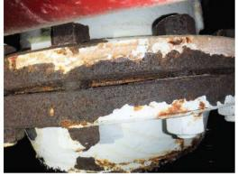
F12) Finding: There is heavy corrosion on the conduits and fittings associated with (5) (3) (A) MOV may fail to operate properly if the corrosion on the conduit damages the internal wiring. Location (b) (3) (A)
