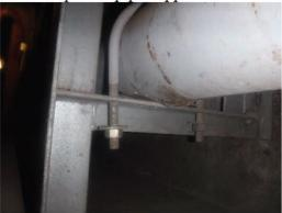
E51) Several locations with lose U-bolts, displaced Teflon pads, missing Teflon pads or loose hangers were noted. Some of the locations are summarized below with a full list to be provided in the report.
