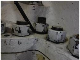
C6) **Finding:** Pump (b) (3) had a skillet installed on the discharge side of the pump nozzle. The assembled joint only had one gasket installed. Similar condition noted on (b) (3).
