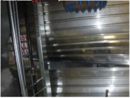
F26) **Finding:** There is no hold down u-bolts or slide-guide to prevent lateral pipe movement at the end of the header pipe run (at (b) (3)
