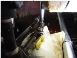
C31) One slightly loose joint harness was noted on the discharge side of pump P-209. Gaps measured between harness lug and nut were approx. 0.030" (enough for the rod and bolt to move laterally).
