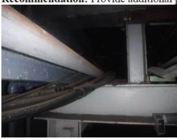
E16) **Finding:** Section of FOR piping from Sump 7 routes through the electrical room. Section of this pipe is not equipped with Teflon pads (metal-to-metal contact).
