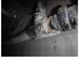
E13) **Finding:** Section of the wall mounted pipe by door C has a wood shim between pipe and support. Note: pipe is not secured to the support.
