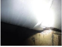
D2) Finding: Deteriorated grout noted at the bottom of the pipe support at (b) (3) (A) (just past the (b) (3) (A)
