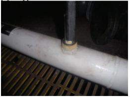
E2) Missing Teflon pad (metal-to metal contact) between pipe and support on Tank 20 FOR line in the trench past tank sampling line branch.
