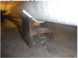
E5) Displaced pipe support on piping within trench between
