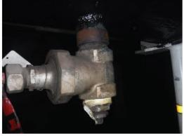
A11) Facility piping at the tank tees has nonstandard (No ASME B16.5) rated flanged fittings and non-standard weld tie-ins. Noted throughout the facility (tees between tanks). Tank 13/14 shown.
