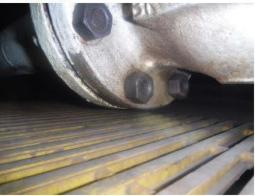
E24) Tank 15 sample lines are not equipped with skin valves positioned as close as practical to the tank shell (and or nozzle).
