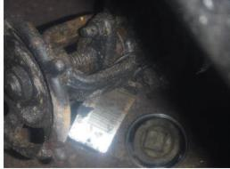
B4) **Finding:** Some staining and wetting were noted on the threaded LPD assembly on (F-76) LPD just past (b) (3) 0 (note the drip pan).
