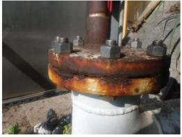
E60) Excessive vegetation around pipe (section of FOR pipe to Tank 311).
