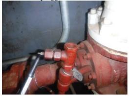
E47) The valve above the FOR isolation valve has a lose flange with several missing
