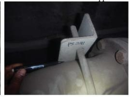
isolation valve to the ADIT 3 door is E49) Segment of tunnel piping from the constructed with mechanical coupling (Style 77 Victaulic joint). Some discoloration corrosion cell and staining were noted at some joints (locations will be identified).
