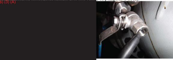
C10) Weeping at suction side pressure gauge associated with Pump P-201.
