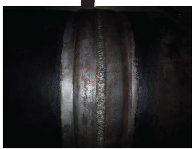
E.70 Typical bell-bell welded with coating removed (Welder ID stamps noted at welds)
