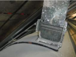
A32) **Finding:** One joint harness with gap ted on the (F76) dresser coupling at (b) (3). There are no deflection rings and adapters on the harness lugs. Note: Eight out of the sixteen lugs are installed backwards (those on the bulkhead side).
