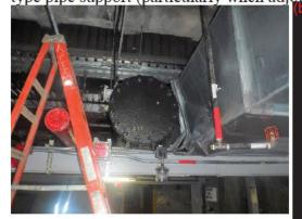
F27) **Finding:** There is coating damage at pipe repair sleeve located approximately 2.5
