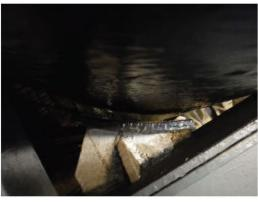
A23) The second pipe support from Tank 9 for the pipe is not in contact with the pipe (floating pipe). It is 39-feet of unsupported pie from tank to the tee.
