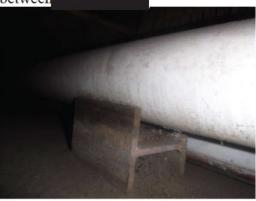
E40) Missing Teflon pad (metal-to metal contact) between pipe and support on FOR line between [NO PHOTO]
