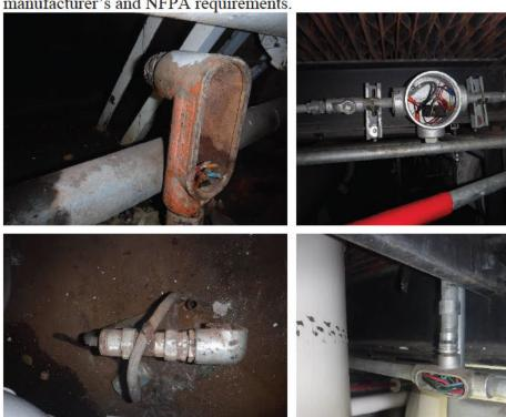
C35) Finding: The open conduit on the UGPH floor will limit the secondary containment capability of the UGPH (no secondary containment).
