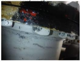
D6) Some staining noted on the bottom of the flange for the JP-5 line from Surge Tank 2; just before pipe support JP5-3 (no active weeping noted). *Note: See comment in Item 5 above about non-fuel related oily material.*
