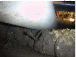
E9) **Finding:** The top of flange just before the FOR concrete pit; Sump 7 (near Door C) is covered with concrete to include side of the flange, face of flange, and fasteners.
