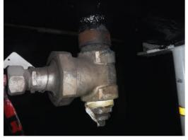
A13) **Finding:** Facility piping at the tank tees has nonstandard (None ASME B16.5) rated flanged fittings and non-standard weld tie-ins. Noted throughout the facility (tees between tanks). Tank 13/14 shown but typical at each Tee at this facility. ASME B31.3 Paragraph 304.7.2 allows "Unlisted Components" provided engineering analysis is conducted and meets one or more of the means stated in subparts. (a) through (d).
