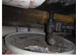
B5) **Finding:** The (b) (3) (JP-5) line just past 690 and before UGPH bulkhead has a threaded LPD. There is notable corrosion on the pipe nipple (red arrow).
