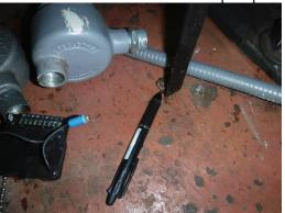
C4) **Finding:** Several open conduits and s or enclosures noted on pump (b) (3) (pump appears to be undergoing repair).
