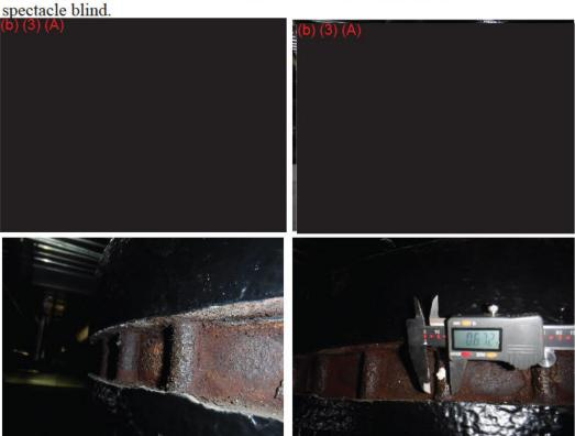
A27) Finding: The branch piping on (6) (3) (F-76) header has a welded and flanged branch fitting at about the 2 o'clock position. Two fasteners were not fully engaged. This is located between (b) (3) and (b) (3) (approximately (b) (3) from (b) (3)).
