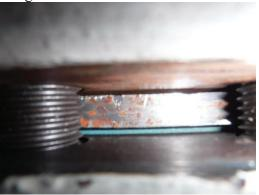
C7) **Finding:** Some minor coating cracks — e noted on the discharge dresser coupling around the middle ring-to-follower joint area of Pump — discharge line (indicating potential movement). This movement is most likely due to loosened joint harnesses and not limitation of the dresser coupling (These couplings have demonstrated satisfactory performance when MFG specification and guidance are followed).
