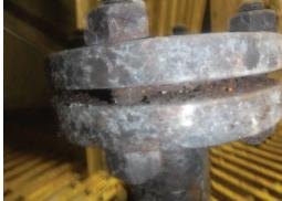
E4) Coating failure and corrosion on the I-beam type pipe supports within the trench (typical throughout the pipe run but noted to be moderate between Tank 20 and Tank 16).
