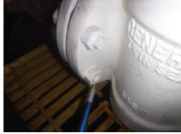
E22) **Finding:** The FOR piping within the trench by Tank 15 has a 2 x 4 wood shim (the support is slanted and not adequately supported).
