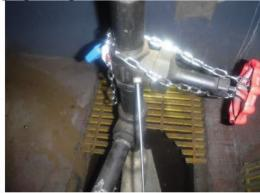
E18) **Finding:** There are three pipe supports in the trench that are displaced near the FOR-line tie-in at Tank 15/16 (past the flange from the above photo).
