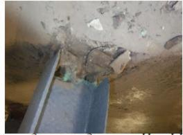
Reference: C/I, Short-Term engaged, wood shim used, saddle not secured to the I-beam. (F-24) line. Note: saddle is not A8) Finding: Pipe not adequately supported at (2) on (2)
