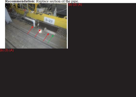
E45) Finding: Several low ultrasonic thickness (UT) data were recorded near the locations where repair clamps are used. A section of FOR pipe was closely checked with a UT gauge, and several locations with thickness ranging from 0.106" to 0.190" were identified indicating over 55% of metal loss was present. The nominal thickness of (b) (3) pipe is 0.237". See next related inspection item.
