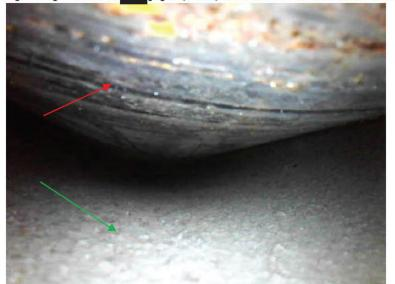
Space between sleeve and pipe. Red arrow is carrier pipe and green arrow is sleeve.
