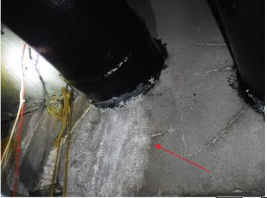
E.18 Efflorescence formation on anchor bulkhead between
