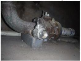
E57) There is moderate coating failure and some corrosion noted on the FOR penetration sleeve just below the ADIT 3 staircase (water infiltration at penetration)
