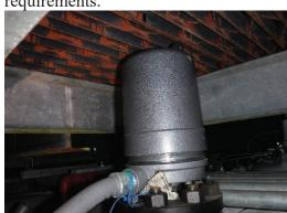
C30) **Finding:** The ½- discharge side pressure gauge threaded fittings have several areas of wetting/weeping around the threaded fitting on Pump (5) (3). Wet absorbent pads noted beneath the fittings.
