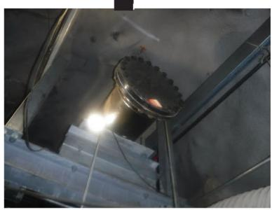
E.25 Unrestrained blind flange at Tank 14 (Tank is out-of-service)
