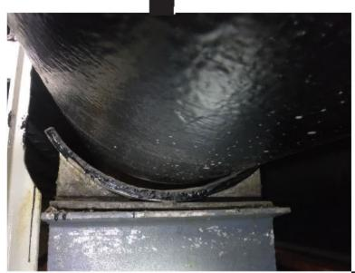
E.16 Saddle type steel support not in contact with pipe at
