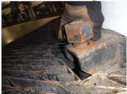
C22) The outlet side flange on the control valve on Pump P-204 is not fully engaged.
