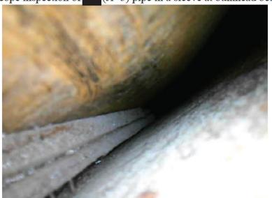
A wood shim was noted between pipe ad sleeve. (Note the nails). LRUT did not indicate corrosion at this penetration but wood shim is not standard practice for sleeve spacer.
