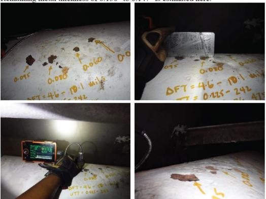
B29) Several inactive pitting and general corrosion on section of the between The pitting/corrosion area is at the 10 o'clock position. Pit depth of 0.080" to 0.140" measured.
