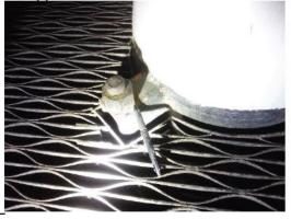
C24) The ball valve before the strainer on the inlet side of the control valve was in the closed position at the time of the inspection on P-205. The control valve may not function as intended when the system cannot detect differential pressure. Consider a car-seal for valve
