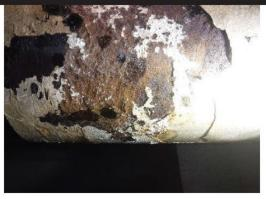
B31) Corrosion on pipe support at the tunnel wall attachment at
