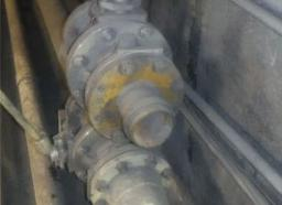
E48) Missing coated U-bolts and isolation Teflon on FOR isolation valves supports.
