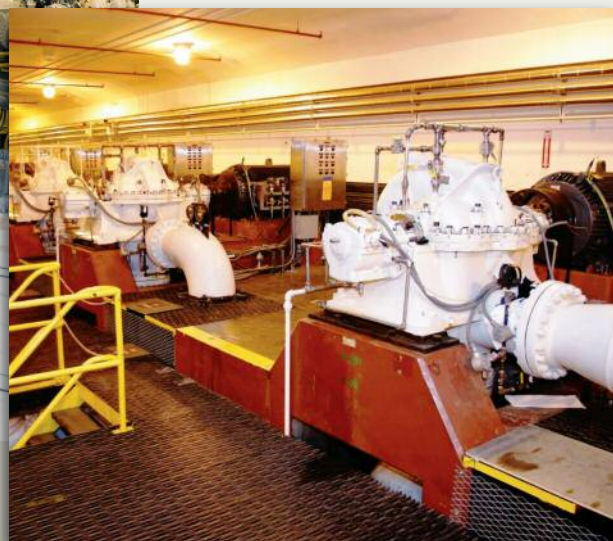
The fuel pumps in the underground pump house.
