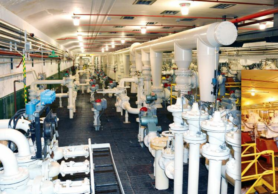
The fuel pumps in the underground pump house.
