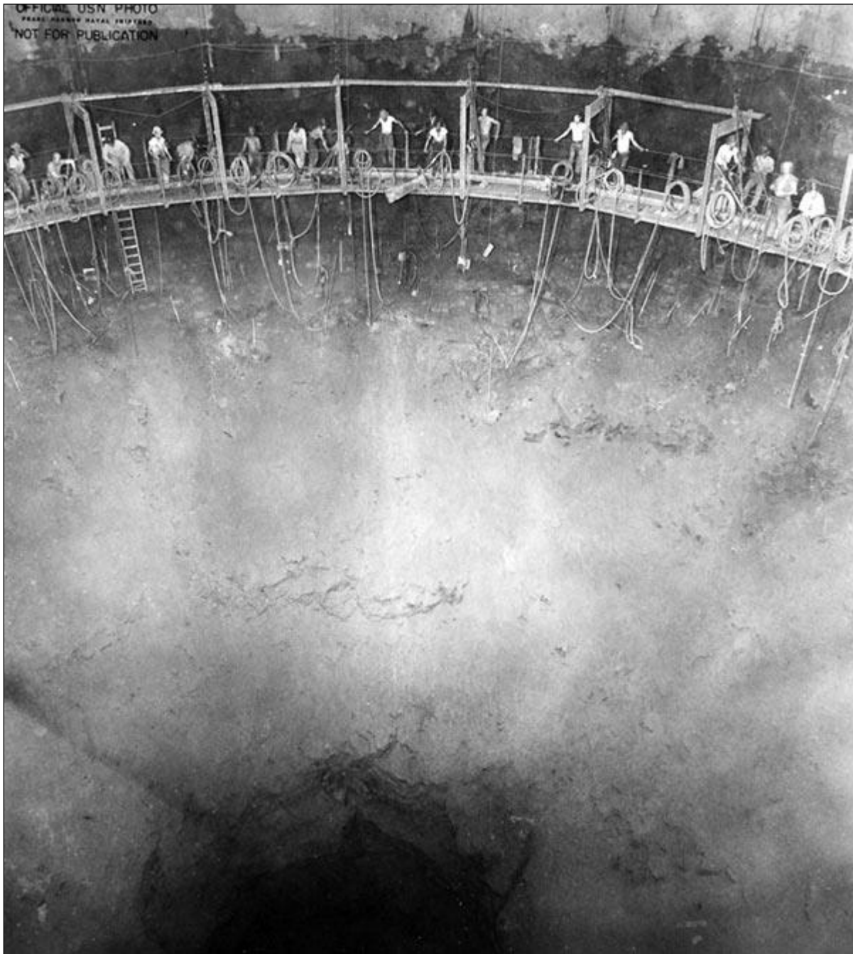
Figure 3.6: Construction of Tank Walls
