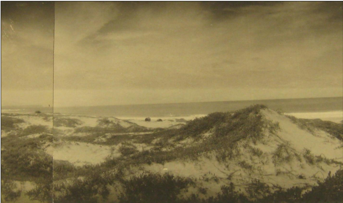
Figure 3.5. Section of 1905 panorama of Barking Sands showing several wooden structures (far left and center) on the makai (ocean) side of the dunes (Hawaii State Archives, Photo Album 19-6).
