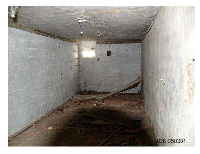
Interior of CP at Dillingham Airfield. Interior dimensions were:  $21'\ 0"\ x\ 9'8"\ x\ 8'0"$  with walls approximately one foot thick. Note rebarrungs ascend to escape housing at the left rear. (Photo by author)
